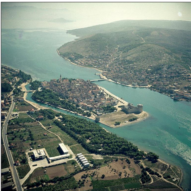
Figure 15: The Trogir motel as an extension of the Adriatic Highway, with the historic town centre in the background. Used with permission from the HDA.
