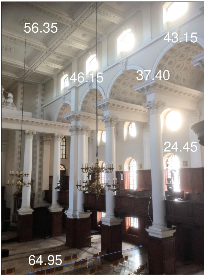
Figure 3: Christ Church. The nave with the south arcade and the coffered vaults, showing significant dimensions marked in feet. The square and cross-shaped (centre left) column pedestals can be seen, and the side wall pilasters supporting the broken entablature from the rear. Photo: Jonathan Hales, 2022.
