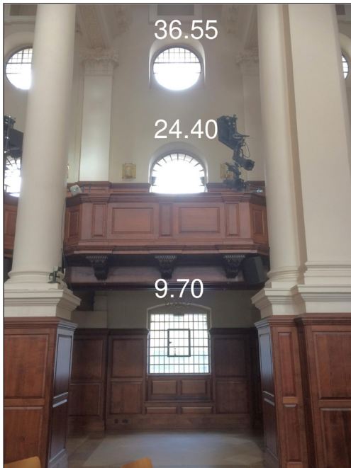
Figure 9: Christ Church, detail of the north wall, showing the side aisle windows, the long windows and the round windows above, with their heights marked in feet. The side pilasters can again be seen, framing the windows and supporting the broken entablature. Photo: Jonathan Hales, 2023.
