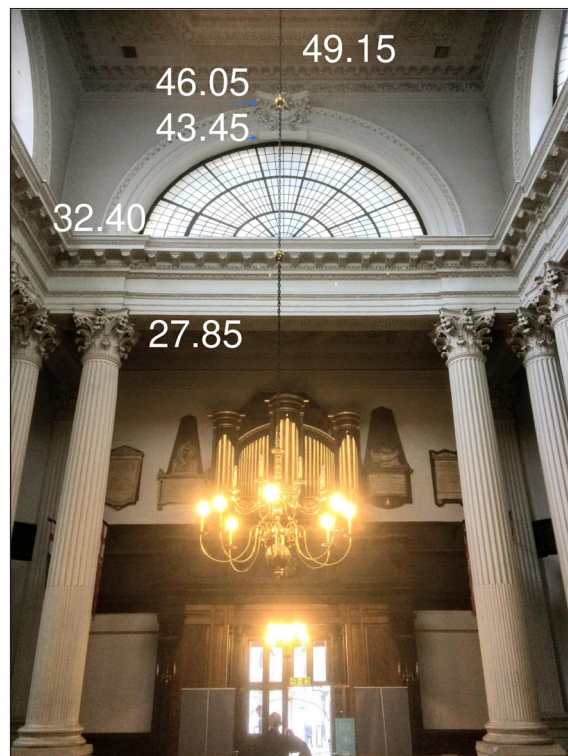
Figure 19: St Mary Woolnoth, the nave looking towards the west entrance, showing the height in feet of significant features. The inner edges of the colonnade pedestals can be seen at the bottom. Photo: Jonathan Hales, 2022.
