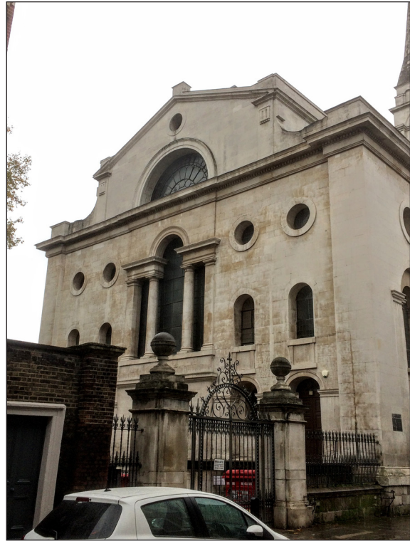
Figure 10: Christ Church, the east façade. The north side door, and the string course visible to the right of it, indicate the nave floor level. Photo: Jonathan Hales, 2022.
