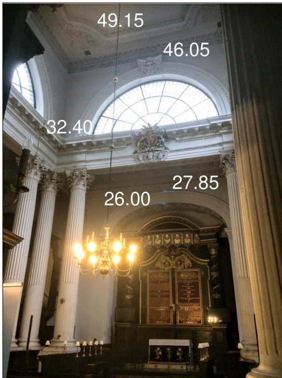
Figure 13: St Mary Woolnoth, the nave looking towards the east end, showing the height in feet of significant features. Masonic imagery is evident in the cherubim on the main entablature below the Royal Arms, and in the glazing bars of the lunette window that evoke the rays of the rising sun. Photo: Jonathan Hales, 2022.
