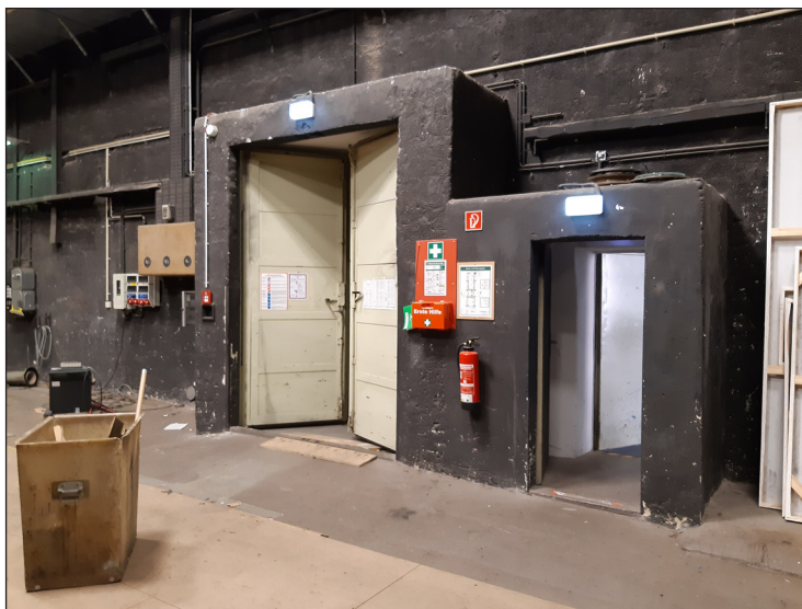
Figure 13: A smaller door for personnel was added at a later stage. Photo by Eleanor Halsall.
