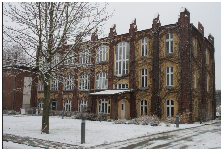
Figure 3: The building in Nowawes that became Ufa's administrative headquarters after Deutsche Bioskop merged with it. Kohtz's Trickfilmatelier (animation studio) is visible to its left. Photo by Eleanor Halsall.
