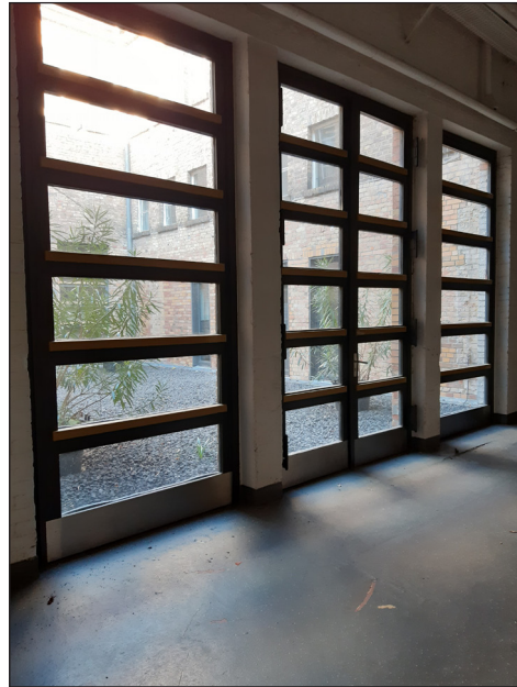
Figure 11: Interior windows. Photograph by Amy Stone.
