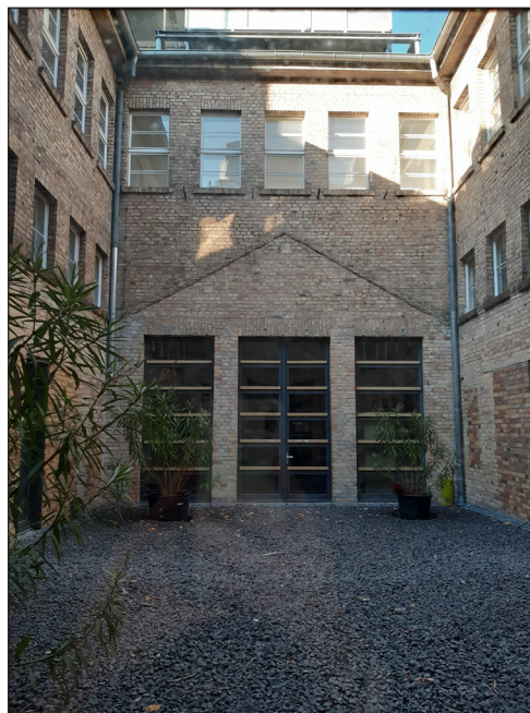
Figure 14: Recent photograph of the inner court. Photograph by Amy Stone.
