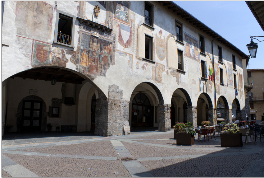
Figure 1: Communal palace, Clusone, south façade.
