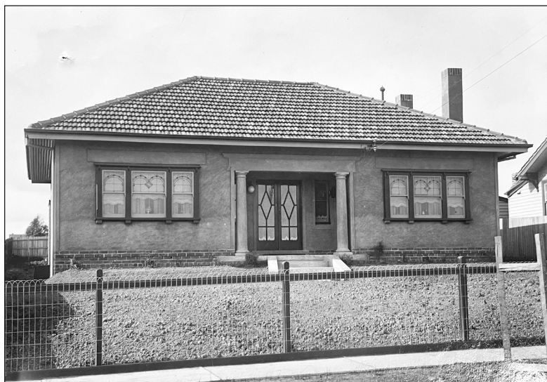
Figure 3: Type B-10, constructed in 1930 for a total cost of £1221/17-. Photograph by Laurie Richards, 1952. Source: Public Records Office Victoria.
