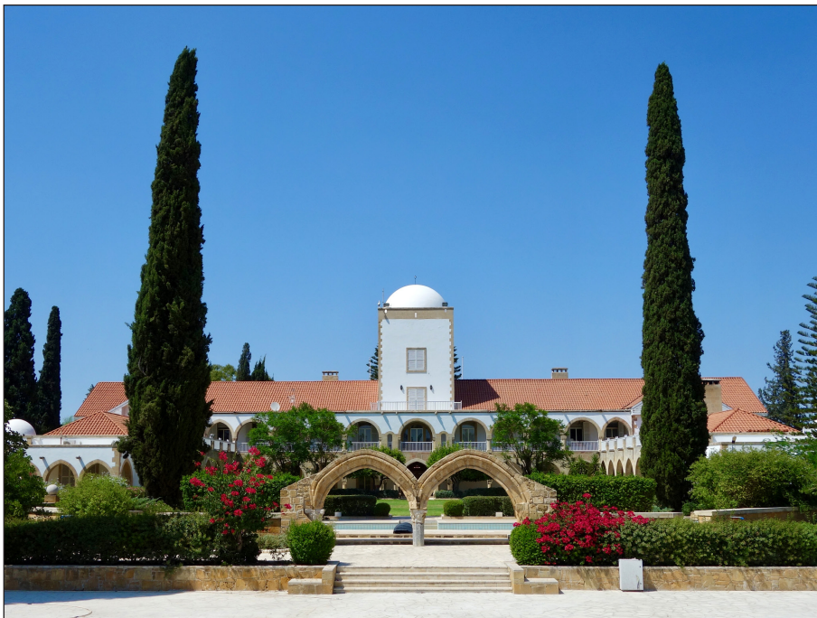
Figure 24: The rear of the new Government House in Nicosia, Cyprus, by Maurice Webb, 1937, featuring arches taken from the city's razed Lusignan Palace. Photograph by Daniel E. Coslett, 2019.
