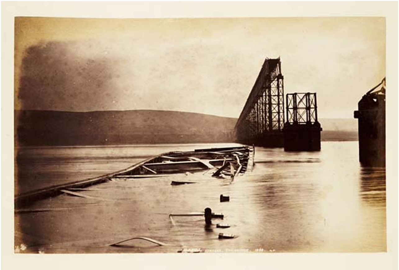
Figure 4: Photograph of fallen girders after collapse of part of the first Tay Bridge, 1879. Reproduced under Creative Commons License from the National Library of Scotland Digital Gallery.
