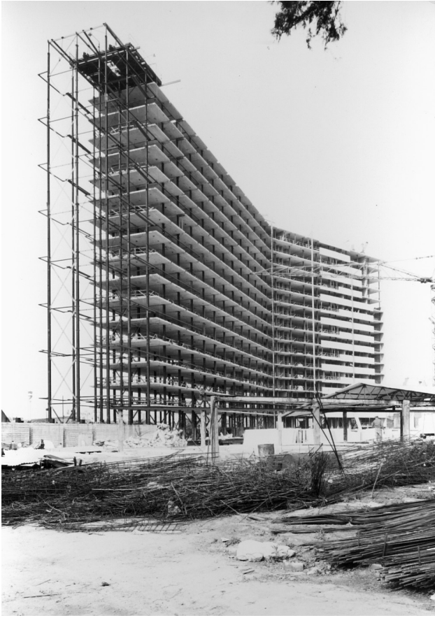
Fig. 3: Close to the collapsed tower stands the incomplete structure of another building on the boulevard Lefebvre estate, which was also being constructed using the 'self-lift' technique. Photo: Coll. Pavillon de l'Arsenal, cliché DUVP 16000, 14 May 1964.
