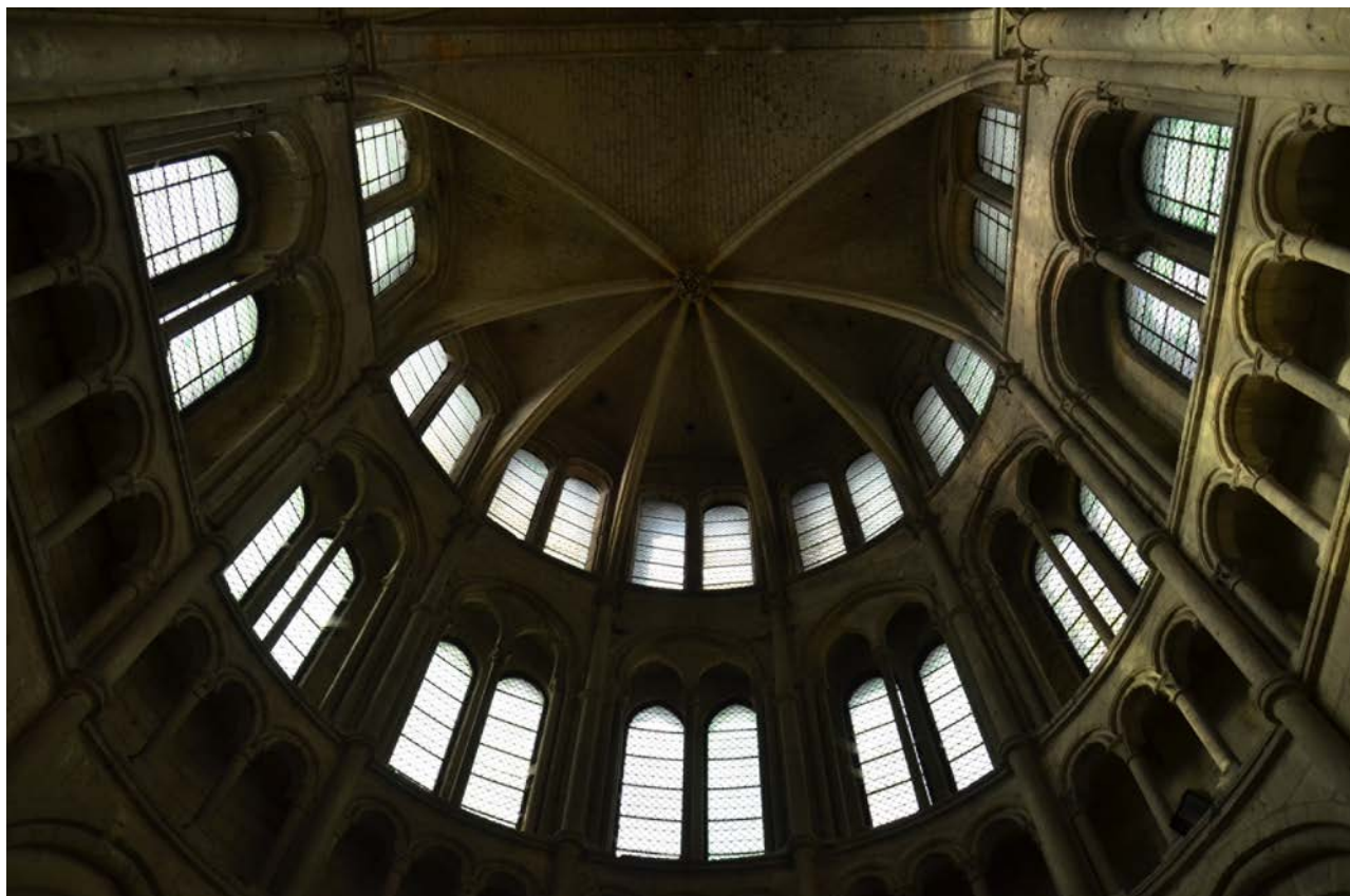
Fig. 8: The south transept clerestory of Noyon cathedral. Photo: author.
