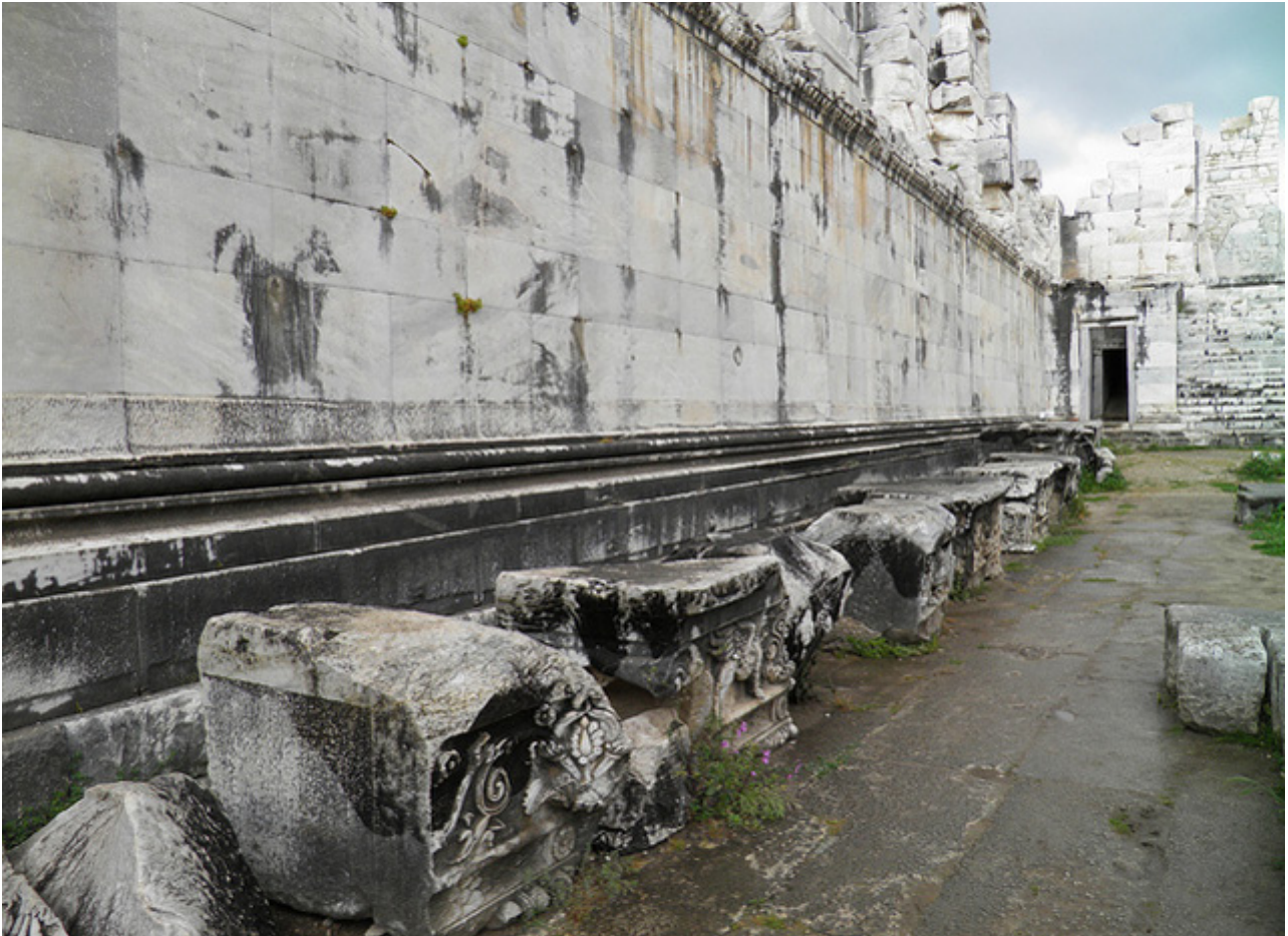
Fig. 5: Photograph of the foundation walls of the Apollo temple at Didyma, containing the construction drawing interpreted in Figure 6 .
