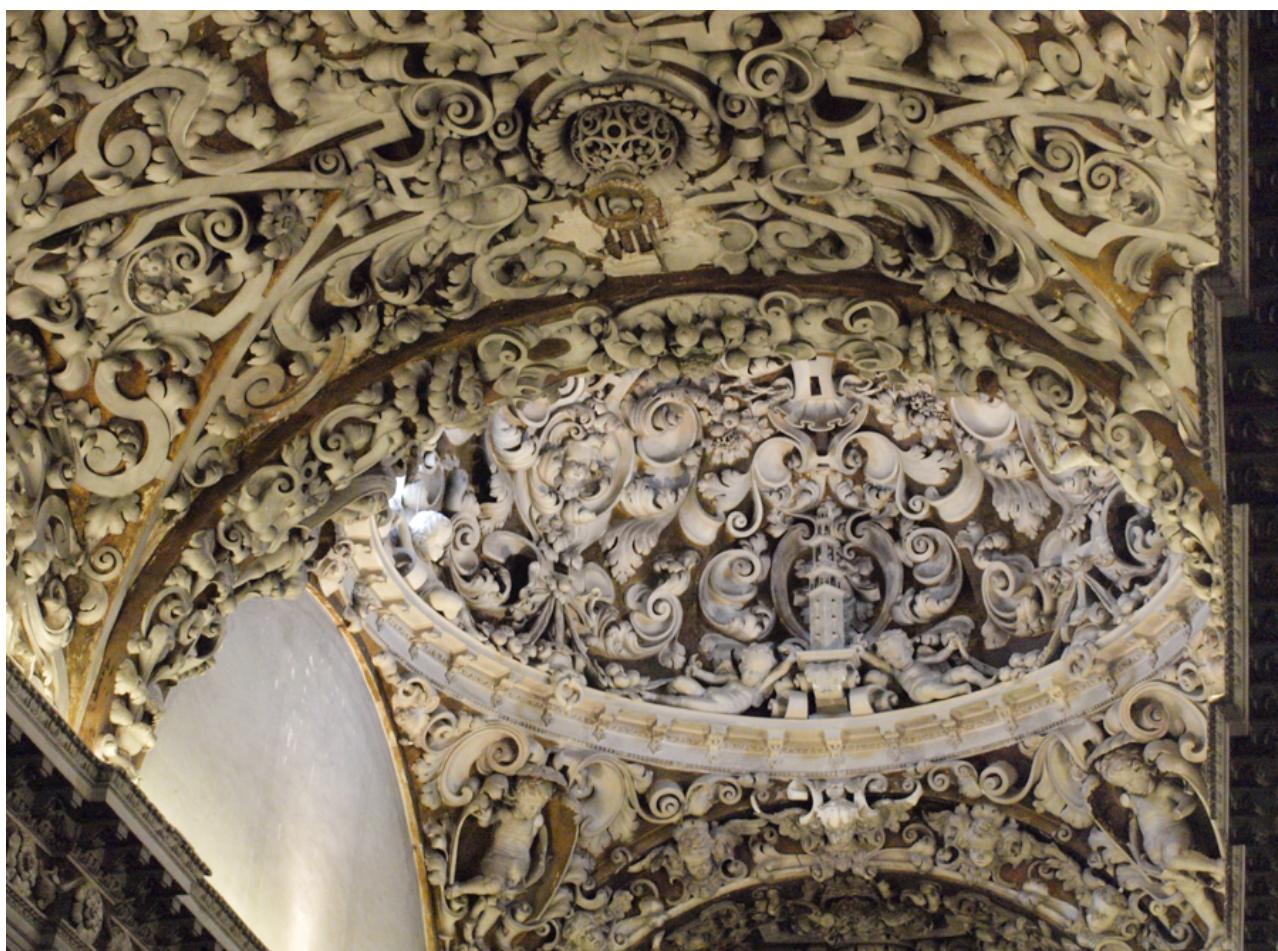
Figure 10: The yeserías on the vaults of the church of Santa María la Blanca, Seville. Image from http://www.flickr.com/photos/isanet/8591929451/in/faves-76073360@N08/ . Photo by Isabel Moguer (Creative Commons license).
