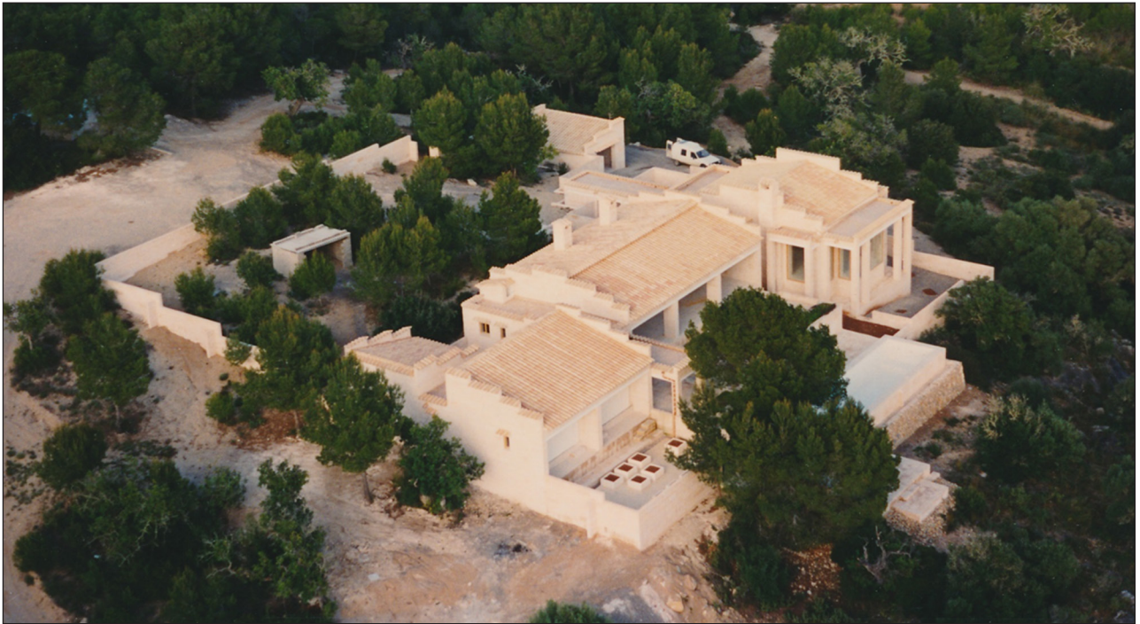
Figure 20: Can Feliz (1994) is built on a podium, its middle pavilion finished with an expanded veranda to create a transitional space between the indoors and the forecourt. Photo courtesy The Utzon Archives, Aalborg University Library.
