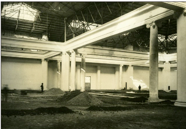
Figure 2: Joan Roig and Emili Canosa. Interior view of the Palace of Textile Industries ( Textilepalast ) under construction. Unknown photographer. AFB, Arxiu Fotogràfic de Barcelona.
