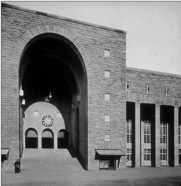
Figure 11: P. Bonatz: Main hall of the Stuttgart railway station, 1914–1928 (Tamms 1937: 20).
