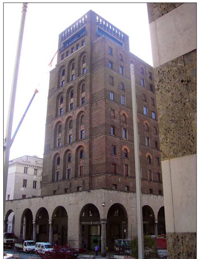
Figure 13: M. Piacentini: INA tower in Brescia (Photo: C. Beese, 2009).
