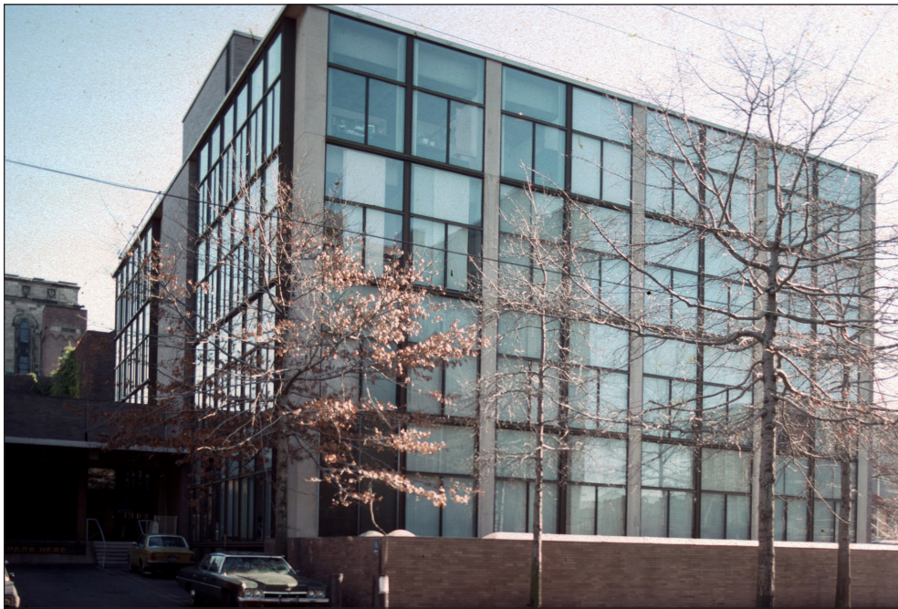
Figure 1: Louis Kahn, New Yale Art Gallery, New Haven, 1951–53, north and west facades, from College Street. Photo by Jean-Louis Cohen, 1981.
