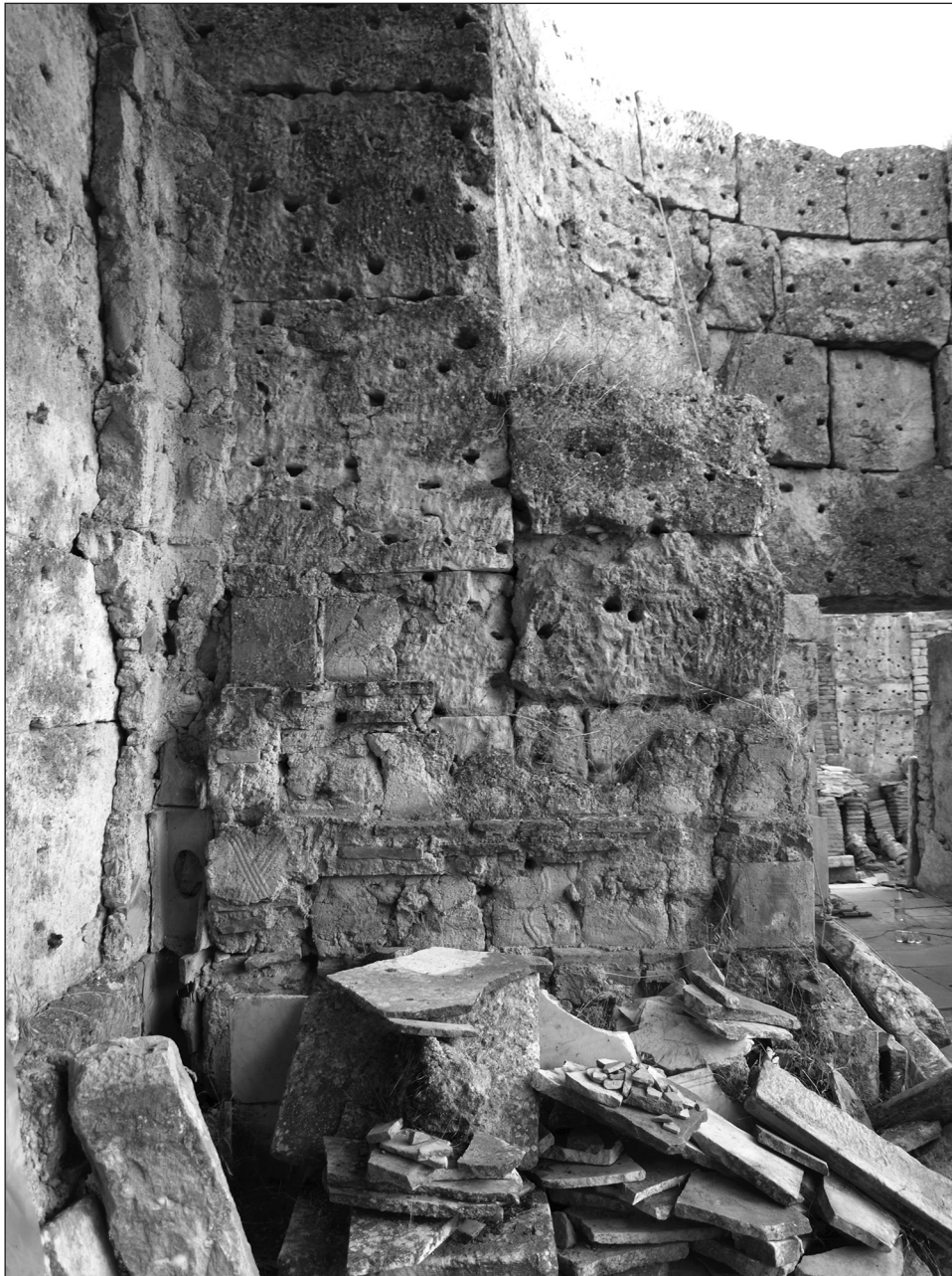
Figure 8: Wall convection system. Hadrianic Baths, Aphrodisias. Photo by A. McDavid.
