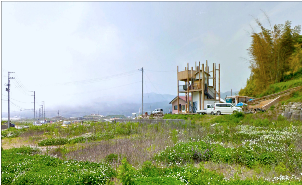
Figure 9: Home-for-All Community Center, Rikuzentakata, 2012. Itō Toyō, Inui Komiko, Hirata Akihisa, and Fujimoto Sou, architects. Photo: Google Street view, image capture June 2013, © Google 2019 < https://goo.gl/maps/i7a6hb-hdHUc8VDpT7 >.
