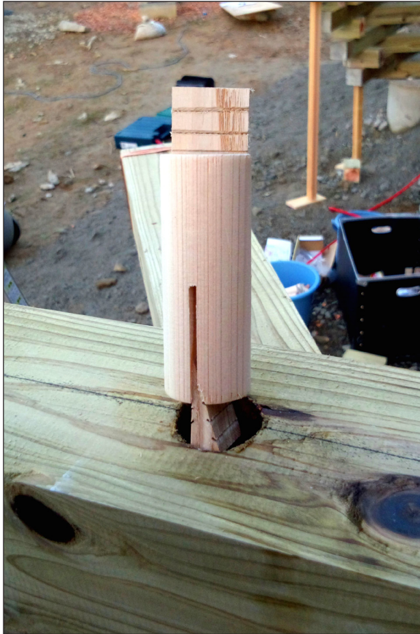
Figure 13: Kozumihama Ojizō-sama Project, Ishinomaki, 2013. Warikusabi split wedge joint detail. Photo by Jun Sato.
