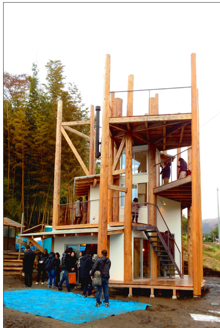
Figure 10: Home-for-All Community Center, Rikuzentakata. Itō Toyō, Inui Komiko, Hirata Akihisa and Fujimoto Sou, architects. Trunks repositioned as structure. Photo by Jun Sato, 2013.
