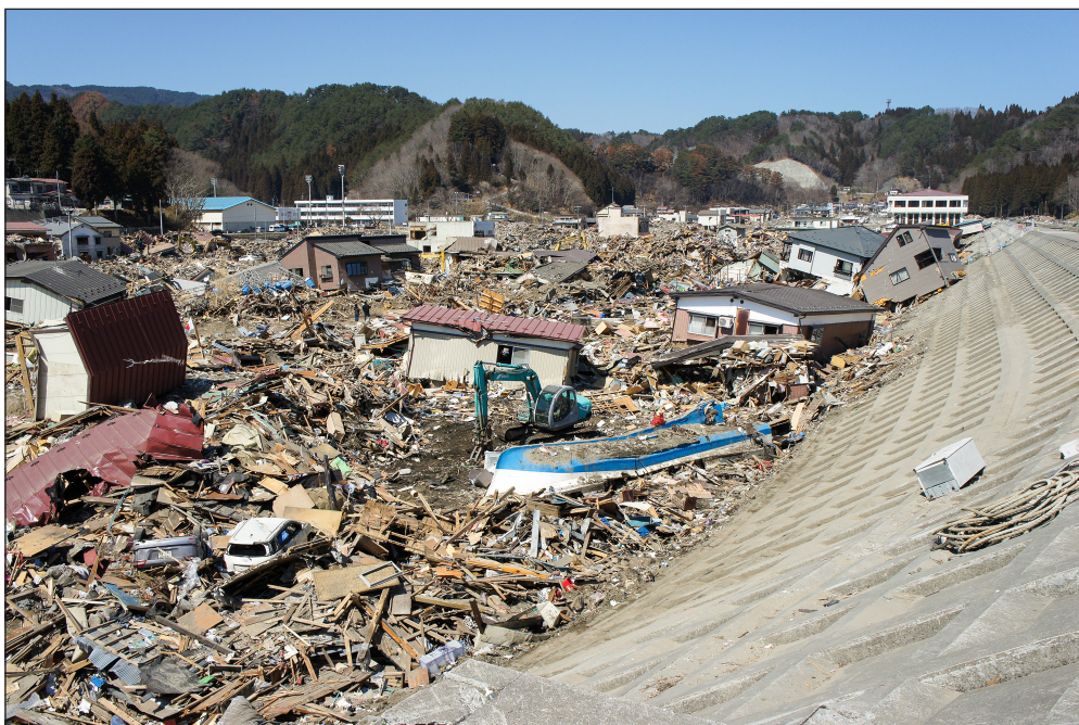
Figure 8: The seawall (on the right) and the devastation in Taro, Iwate Prefecture, on April 6, 2011. Photo by Jim Peterson.
