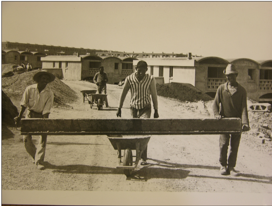
Figure 9: Workers on the construction site at Oued Ouchaya, Algeria, c. 1964. Cité de l'architecture et du patrimoine/Archives d'architecture du XXe siècle, Paris.
