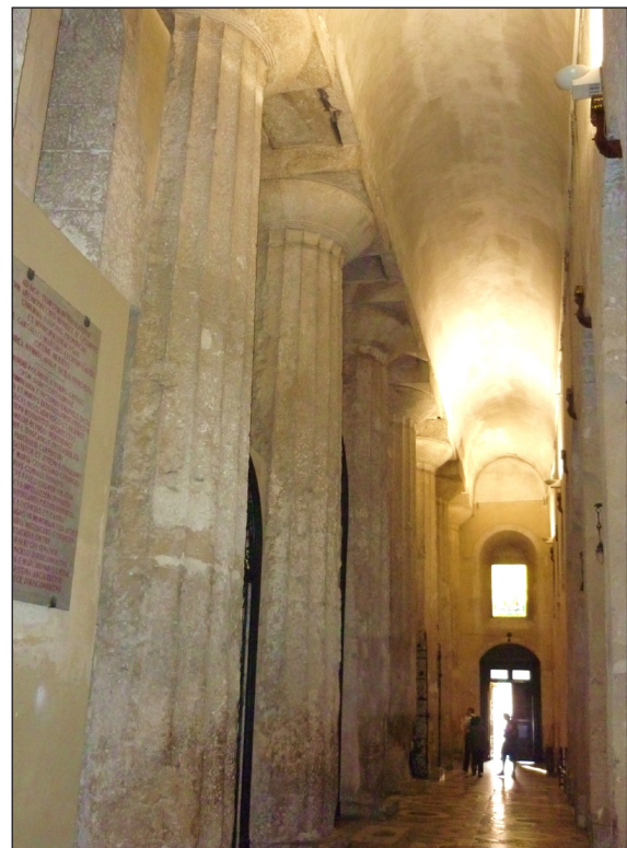
Figure 6: Cathedral of Syracuse, north wall (interior) with integrated Greek columns. Photo by Jo'anne van Ooijen, 2011.
