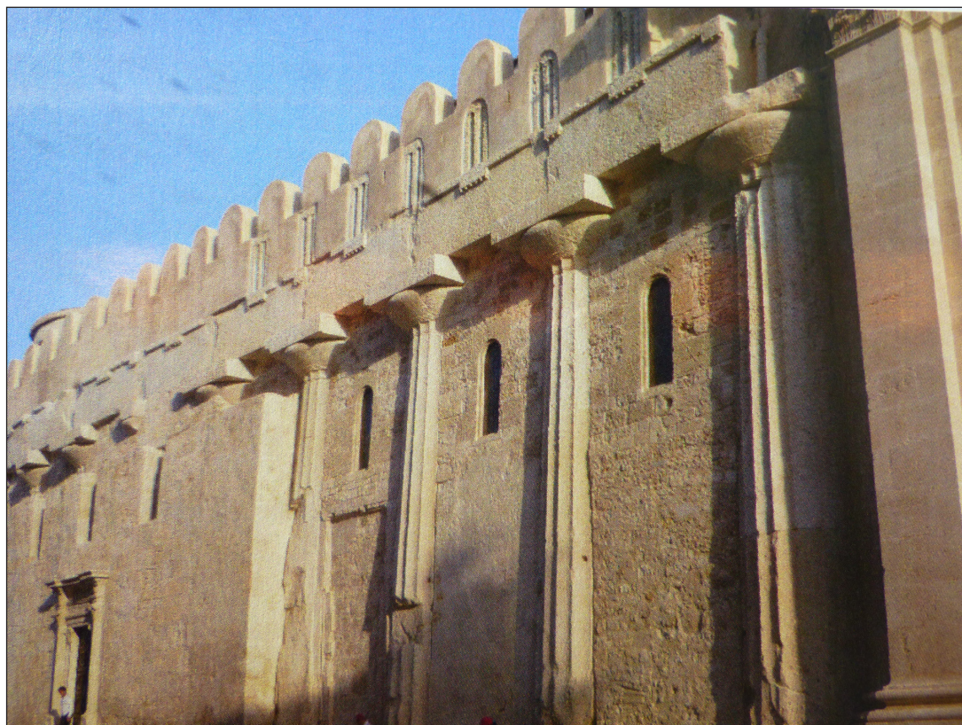
Figure 5: Cathedral of Syracuse, north wall (exterior) with integrated Greek columns. Photo by Jo'anne van Ooijen, 2011.
