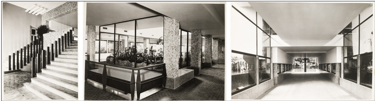
Figure 10: Interiors of the acquario-reptilario , 1960: entrance hall, central corridor on the ground floor and raised crocodile cage. AEV b.20 © Archivio di Stato di Torino.
