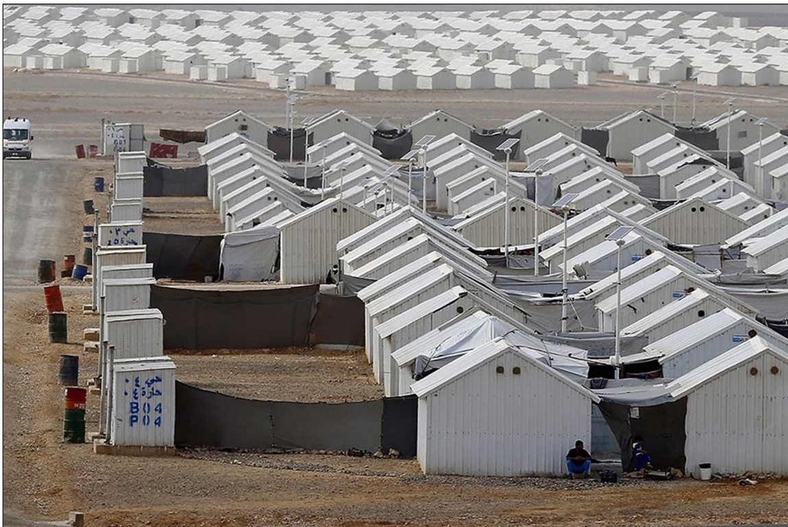
Figure 2: Standardised shelters in Zarqa Camp, Jordan, showing how inhabitants use fabric sheets to provide privacy between households (Davies 2016).
