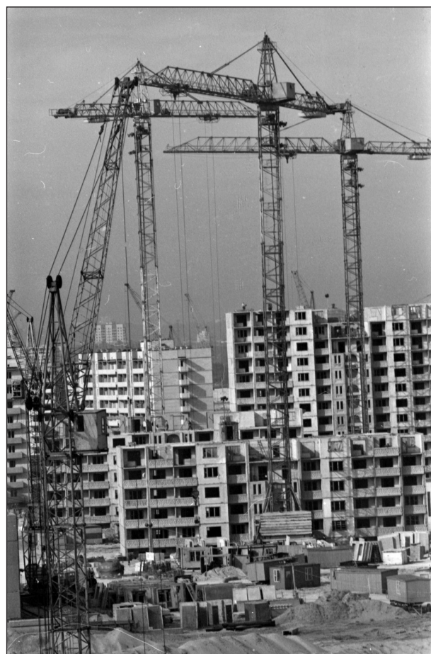
Figure 7: Panel construction in the 1980s: Troeshchina neighborhood of Kyiv, 1983–1984. Courtesy of Tsentral'nyi derzhavnyi kinofotofonoarkhiv Ukrainy im. G.S. Pshenchnogo.
