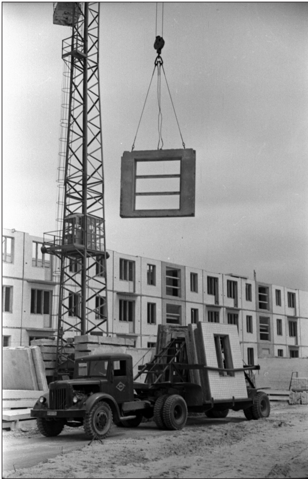
Figure 2: Prefabricated panel construction in 1961 and 1964, Darnytsia neighborhood, Kyiv, Ukraine. Courtesy of Tsentral'nyi derzhavnyi kinofotofonoarkhiv Ukrainy im. G.S. Pshenychnogo.
