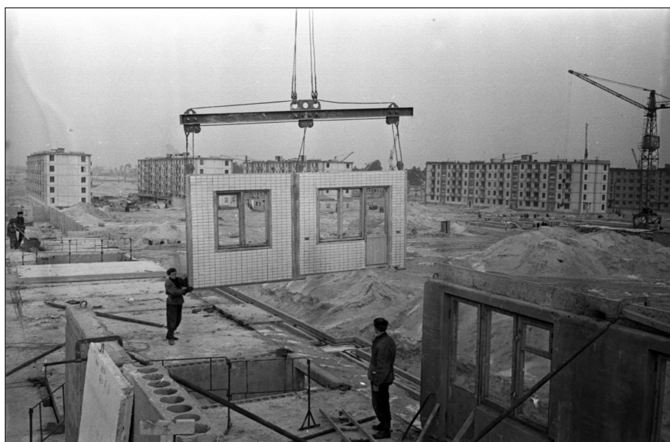
Figure 1: Prefabricated panel construction in 1961 and 1964, Darnytsia neighborhood, Kyiv, Ukraine. Courtesy of Tsentral'nyi derzhavnyi kinofotofonoarkhiv Ukrainy im. G.S. Pshenychnogo.
