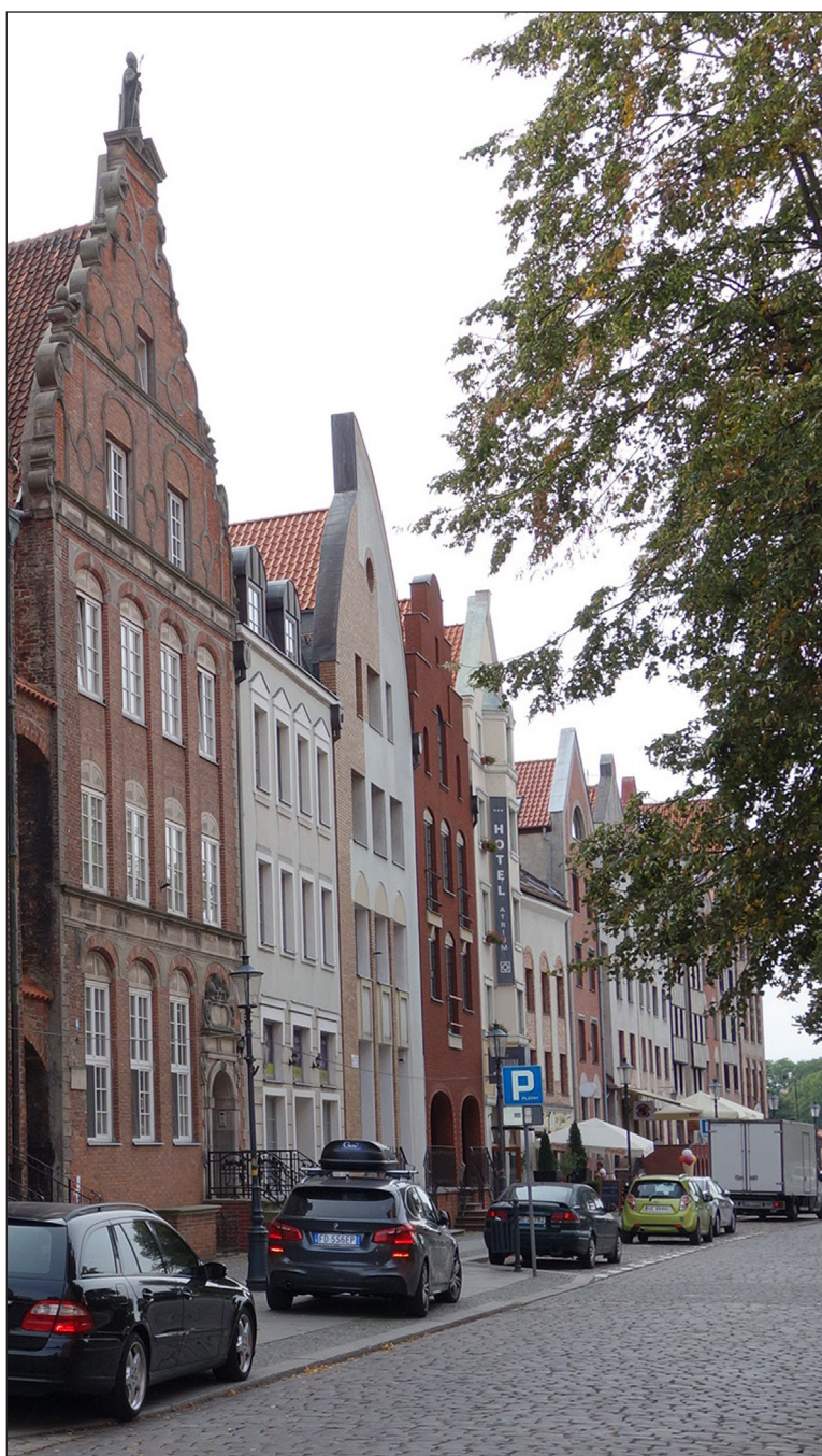
Figure 11: The same view as in Figure 10, in 2018. Only the building Mostowa 17 (left), as well as the adjacent buildings Mostowa 18 and 19 (not visible on the picture; see Figure 12) were rebuilt according to the historical model. Photo by Florian Urban, 2018.
