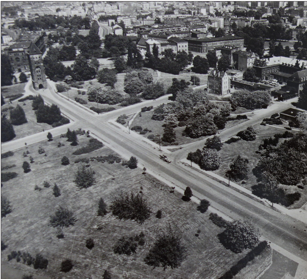
Figure 2: The same view in 1975. The Brama Targowa (Market Gate) is visible in the top left corner (Barton 1975: photograph no. 111 by A. Wołosewicz).
