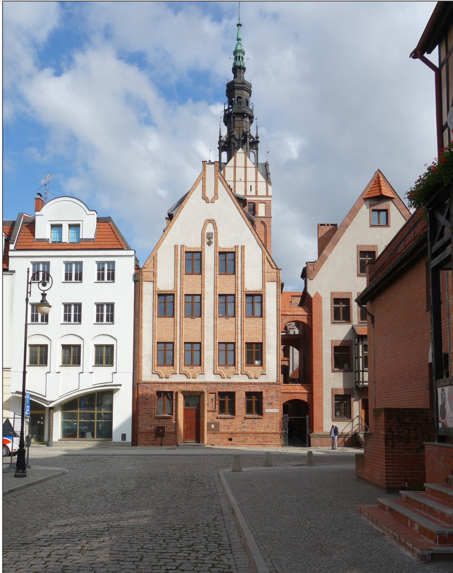
Figure 4: Left to right: The buildings at Świętego Ducha 21, 20, and 19, rebuilt in the 1980s, with the entrance of the Ścieżka Kościelna (Church Alley). The cathedral is in the background. Photo by Florian Urban, 2018.
