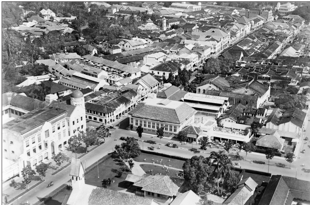
Figure 10: Kesawan, Palace Street and Soekamoelia in Medan (ca. 1930). Tjong A Fie's Mansion is visible on the right side in the centre. (Stichting Nationaal Museum van Wereldculturen, Amsterdam: Inv. No. TM-10015046).
