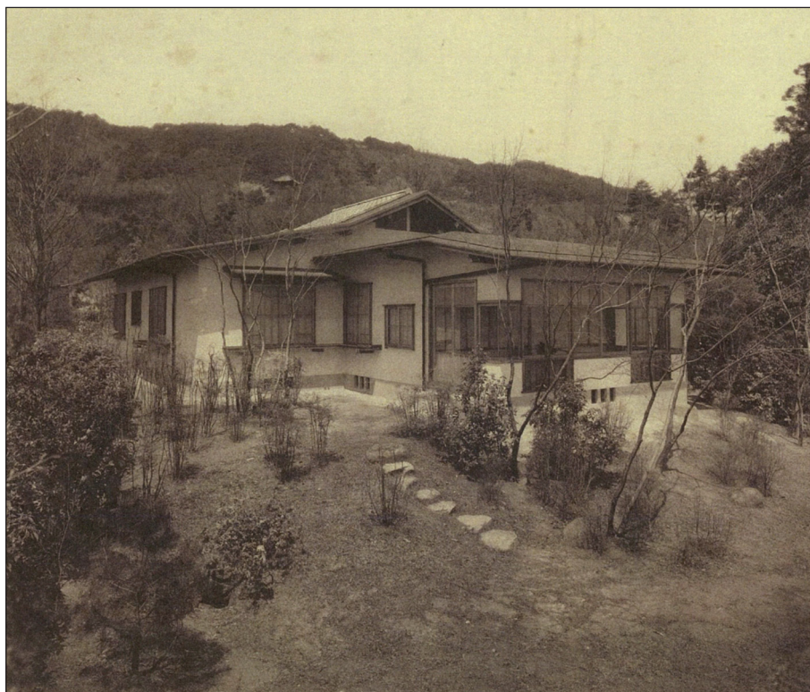
Figure 15: Exterior of Chōchikukyo, Chōchikukyo zuanshū , 1929.
