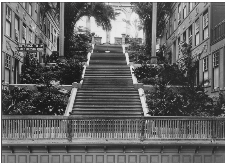
Figure 10: Sutro Baths, view up the grand staircase at Sutro Baths, c. 1900. Marilyn Blaisdell Collection, OpenSFHistory.org/Western Neighborhoods Project, wnp70.0573.
