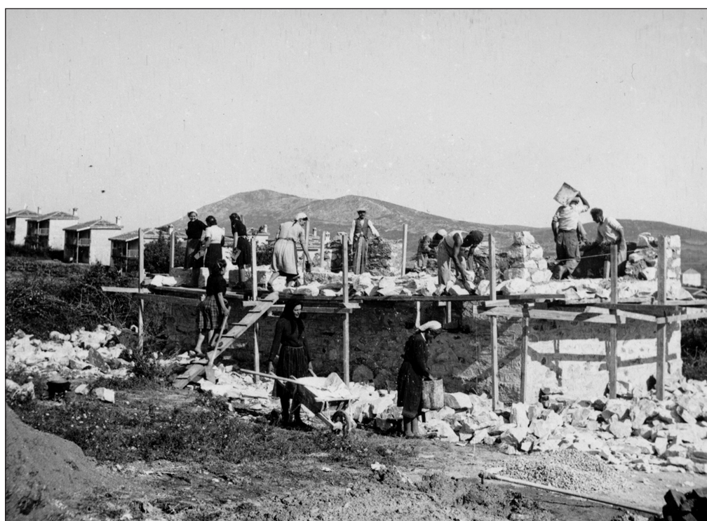
Figure 14: The construction of housing ‘cores’ through ‘self-help’ practices (c. 1949). Kardamitsis archive, Modern Greek Architecture Archives, Benaki Museum.
