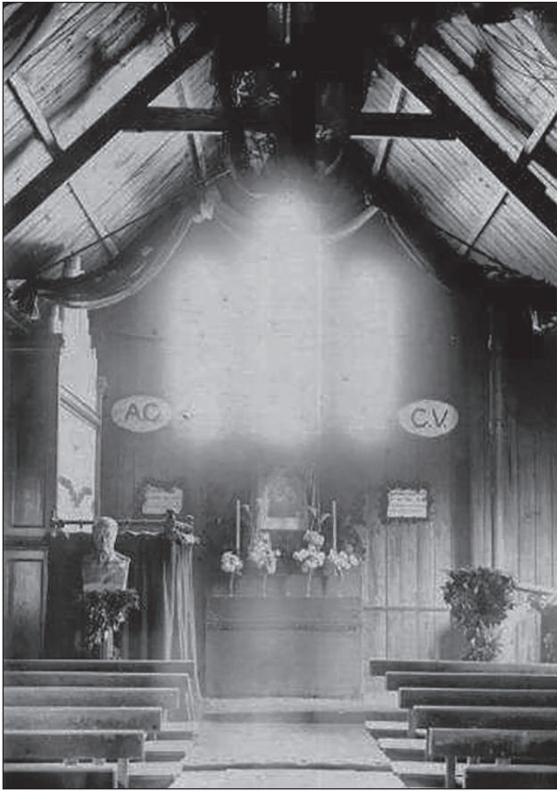
Figure 7: The interior of the demolished Newcastle Temple of Humanity, undated. The letters 'A.C.' and 'C.V.' in the painted signs refer to Auguste Comte and the subject of his unrequited love, Clotilde de Vaux. Courtesy of British Library of Political and Economic Science, London Positivist Society, 5/4.
