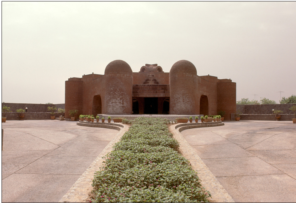
Figure 1: Main entrance of the Belgian ambassadorial residence in New Delhi with its exposed brickwork and lingam-shaped volumes, 1985 (© Massachusetts Institute of Technology, courtesy of Peter Serenyi).
