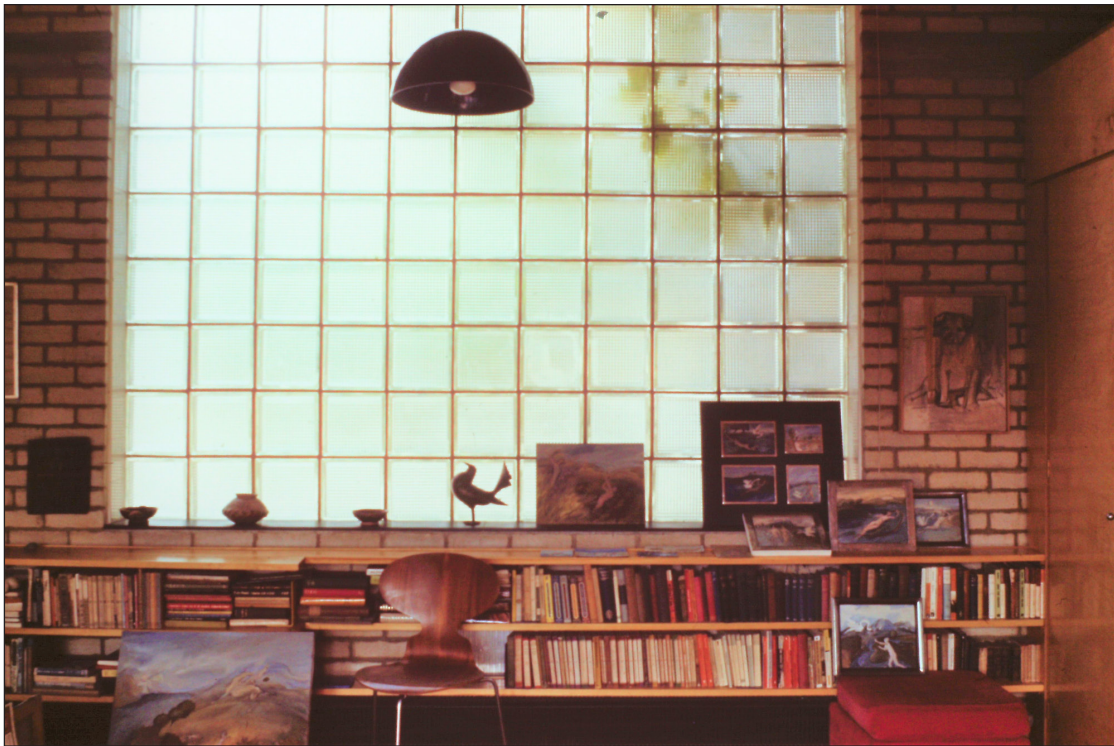
Figure 17: Interior view of Anne's painting studio and the large north-facing glass block window. © Jessica Strang, 1971.
