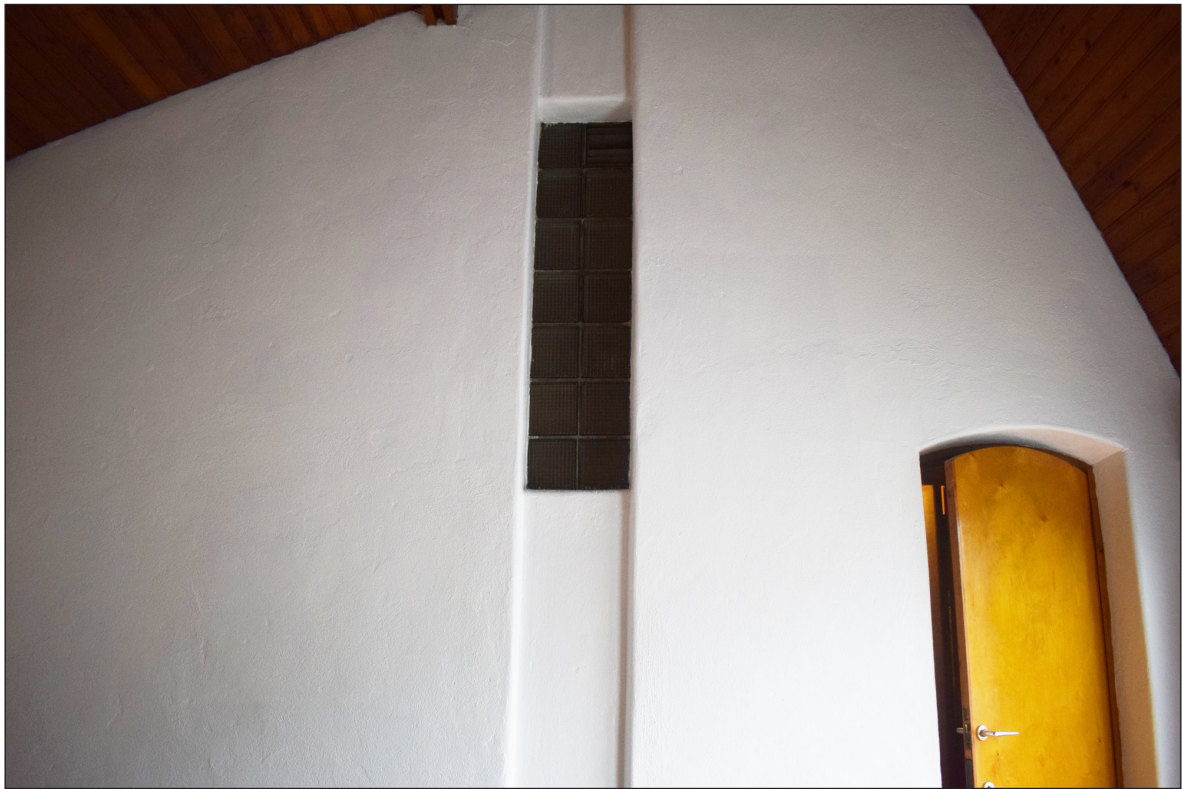
Figure 14: The living room's connection with the original conversion, with the whitewashed rendered wall and rounded reveals. Photograph by Stephen Parnell, 2019.
