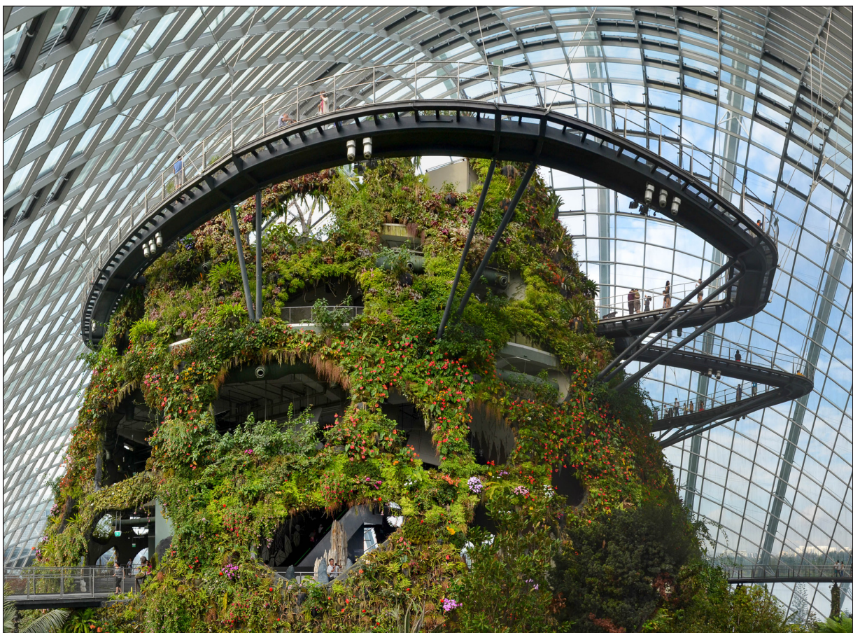
Figure 9: Interior view of the greenhouse with a subtropical climate at the conservatory of the Gardens by the Sea, Singapore. This climate is created by the cooling effect of what is called the Cloud Forest. Photo by Jiati-Hwee Chang.
