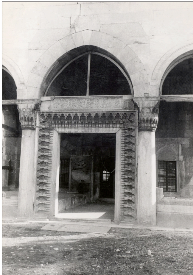
Figure 3: Door frame of the portico with the demolished balustrades. Photograph taken in 1946. ASÚA, SALT. https://archives.saltresearch.org/handle/123456789/78893 .
