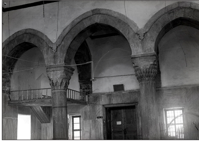
Figure 2: View of the Green Mosque's vestibule with the elevated lodge. Photograph taken in 1938 or earlier: Note the marble column with iron clamps: From Ülgen (1938: R16).
