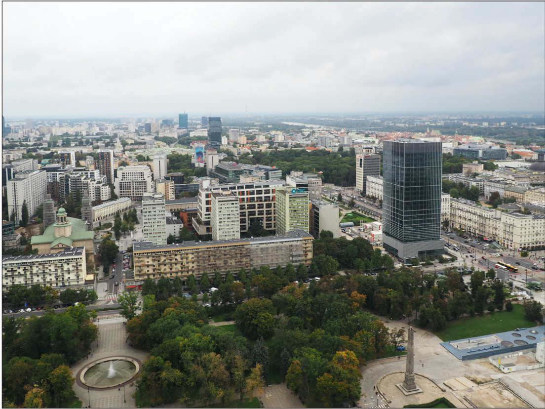
Figure 12: Central Point building on the right, view from the Palace of Culture and Science. Architect: Kazimierski i Ryba, Warsaw. Developer: Immobel Poland. Construction finished: 2021. Photo by Alicja Willam, 2021 © CC BY 2.0.
