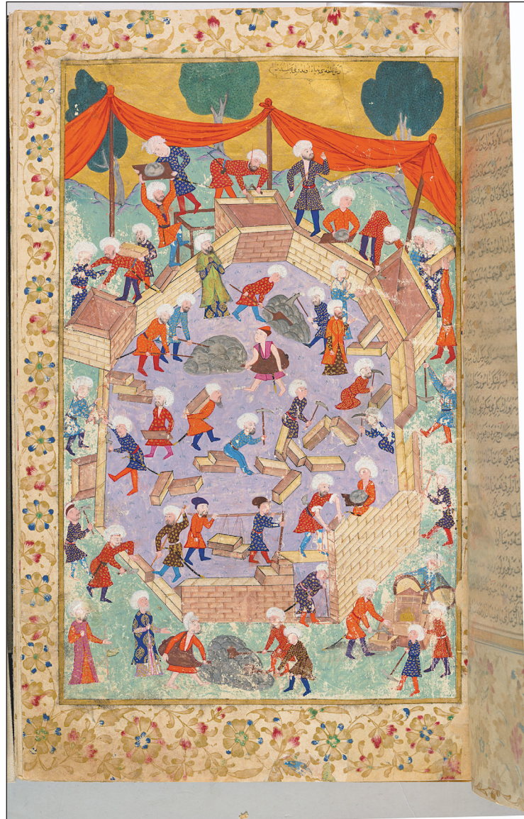
Figure 5: Construction site of the Ares Castle, showing master masons striking stones with pickaxes. Gelibolulu Mustafa Âlî, Nusretname , TSMK, H. 1365, fol. 113r. © Photo courtesy of Topkapı Palace Museum Library.
