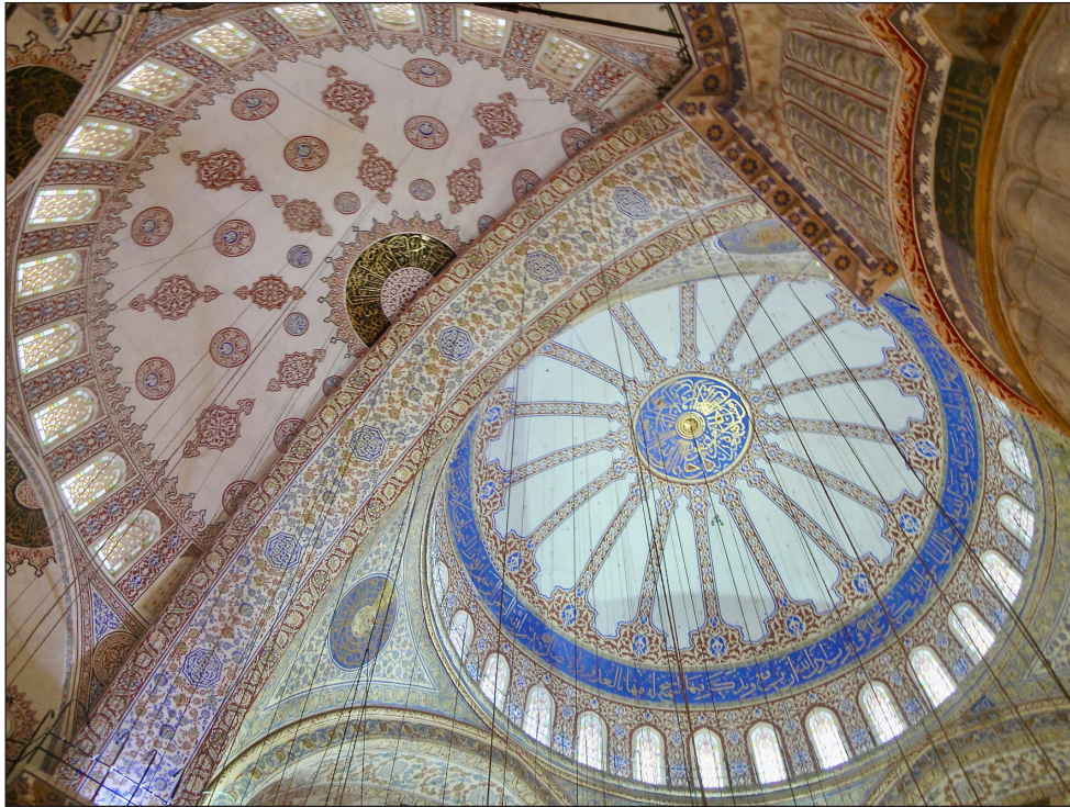
Figure 7: Main arches, pendentives, and drum windows under the dome of the Sultan Ahmed Mosque, 1617, Istanbul. Photograph by the author, February 11, 2013.
