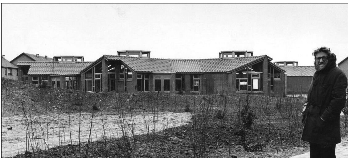
Figure 13: Jan Verhoeven, exterior view of the Cuijk school building in 1976, with Jan Verhoeven in foreground: a building with neither a front nor a back. HNI, Verhoeven, J. / Archief.
