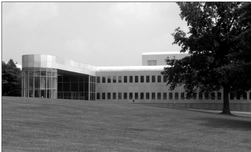
Figure 5: Exterior of COMSAT Laboratories, Clarksburg, MD, built in 1969. © Preservation Maryland.
