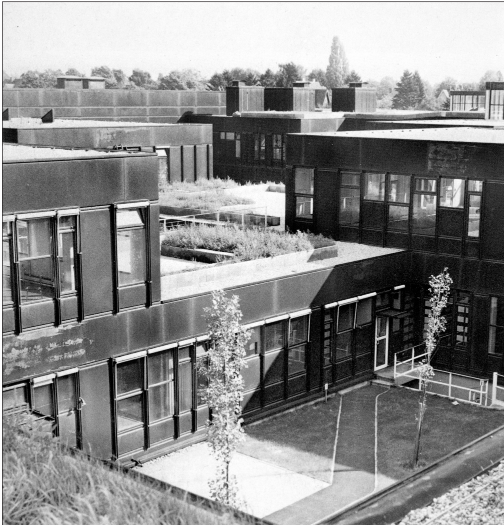
Figure 11: Humanities department building at the Freie Universität Berlin (1963–82), interior courtyard with Corten steel façades, 1973 (Nestler and Bode 1976).
