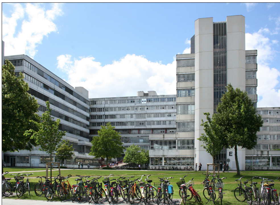
Figure 2: Universität Bielefeld in 2016. During the renovation, the façade will be completely replaced. Photo by the author.
