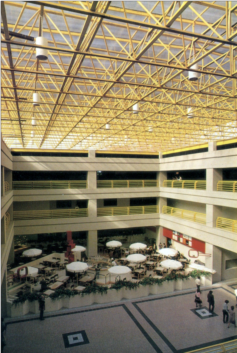
Figure 19: Harley spaceframe used in the International Airport of Mexico City. Edwin Codd, private collection.
