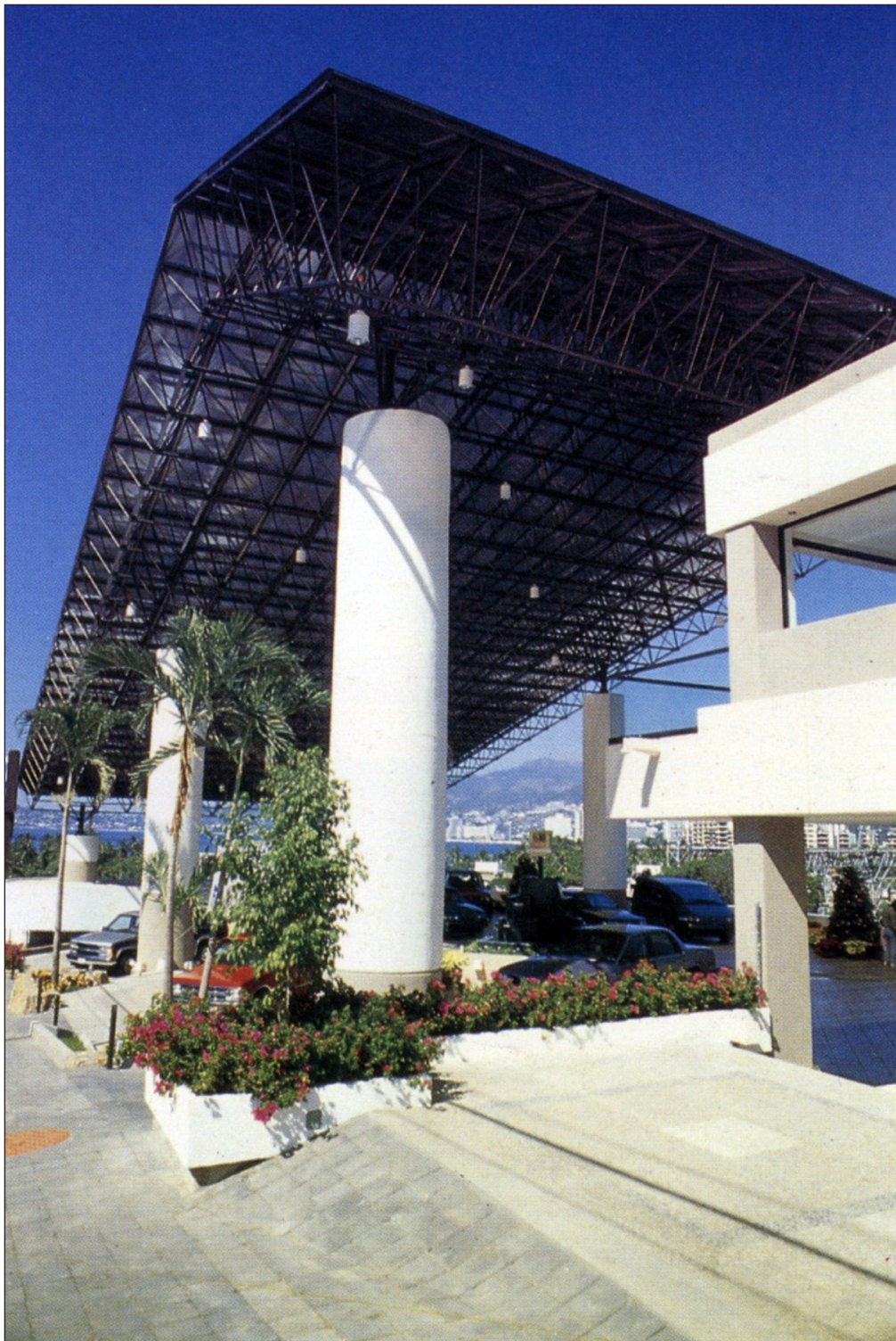
Figure 21: Harley spaceframe used in the distribution centre of General Motors in Acapulca, Mexico. Edwin Codd, private collection.
