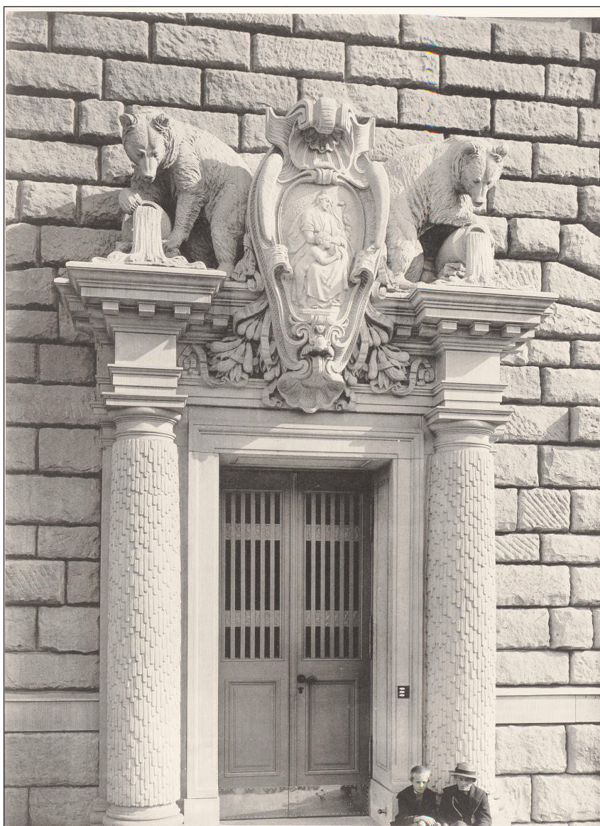
Figure 8: Bärwaldstraße public bath, detail of portal. Sculpture by Otto Lessing. Photograph by Ernst von Brauchitsch, published in volume 1 of Neubauten der Stadt Berlin (1902). Image courtesy of Architekturmuseum TU Berlin, Inv. Nr.: B 2371,030.
