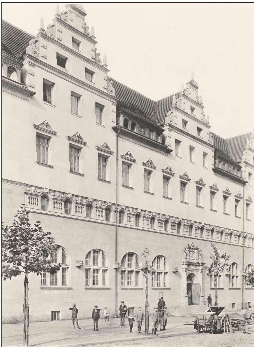
Figure 9: Oderbergerstraße bath, view of façade. Sculptural details by Otto Lessing. Photograph by Ernst von Brauchitsch, published in volume 2 of Neubauten der Stadt Berlin (1903). Image courtesy of Architekturmuseum TU Berlin, Inv. Nr.: B 2372,055.
