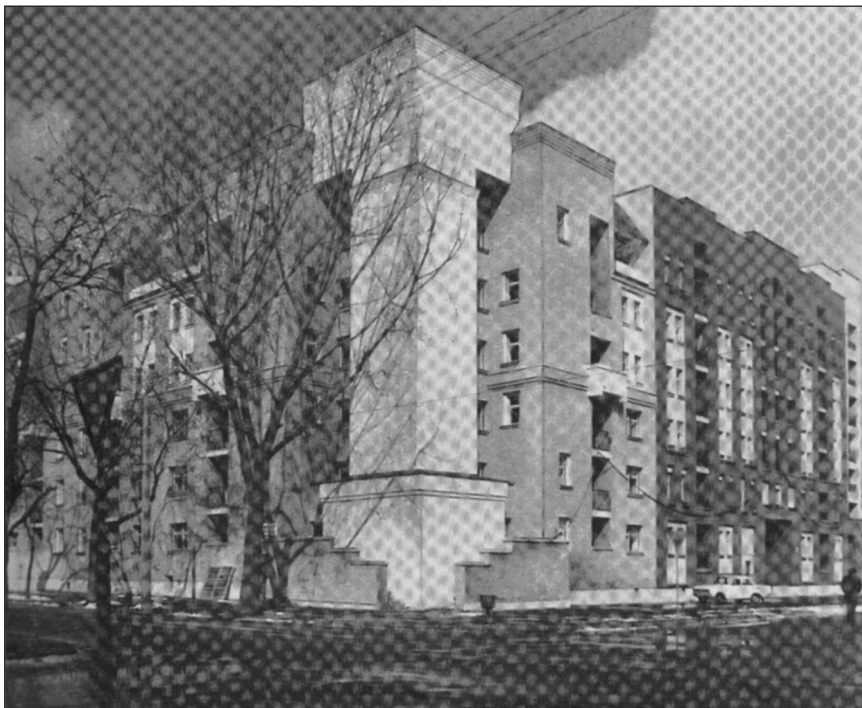
Figure 5: T. V. Lazarenko, Iu. S. Shalatskii and I. P. Shpara, residential block in Podil, Kyiv, Ukraine, completed in 1989. From 'Kvartal V-14 na Podole' (1989: 37).
