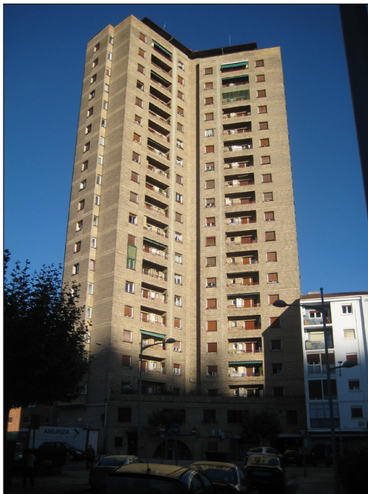
Figure 17: View of the Kurtze Txipi tower (68-Ar), in Arrasate (1968), by Luis Astiazarán. Photo by Lauren Etxepare, 2021.
