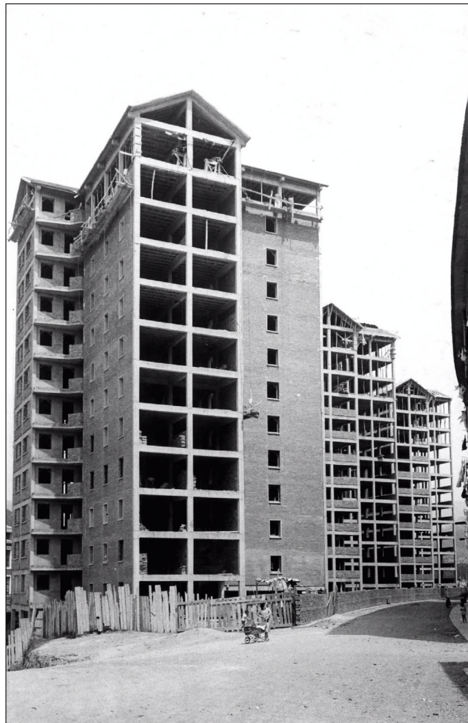
Figure 2: Construction of the structure of the towers in Armeria (59-Ei), in Eibar, built in 1959. Archivo Municipal de Eibar.
