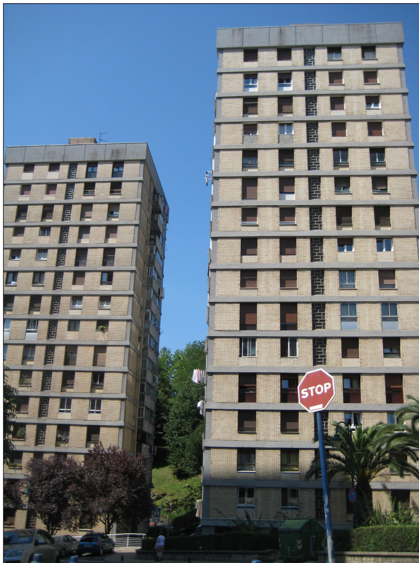
Figure 21: View of two towers of Polígono Capuchinos (70-Er), in Errenteria (1970), by Félix Llanos. Photo by Lauren Etxepare, 2021.
