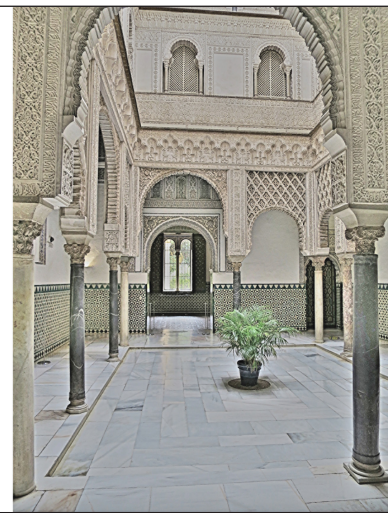
Figure 24: Patio de las Muñecas, photograph taken by the author in 2021. Everything above the ground-floor arch directly ahead is an 1843 invention, as is the ajimez seen through the door.
