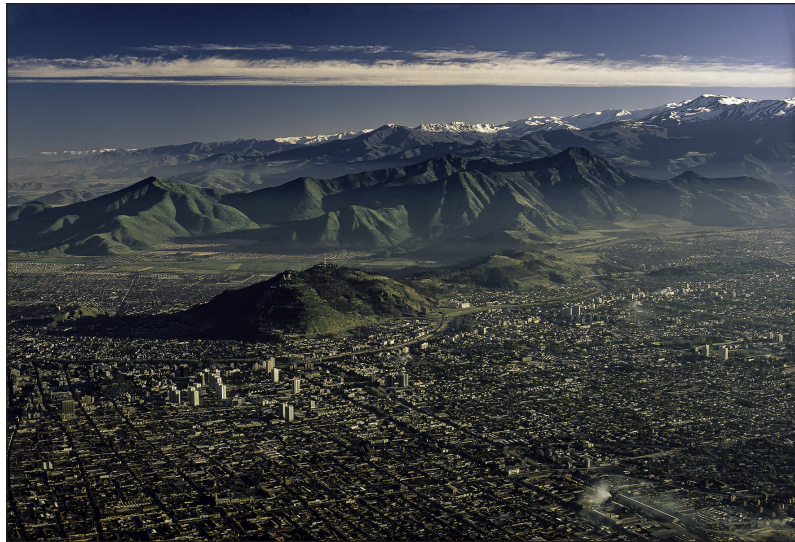
Figure 2: The San Borja Remodeling was the only high-rise complex in Santiago at that time. Aerial view of Santiago, c. 1973. Photo by George F. Mobley for National Geographic Magazine . Young and Mobley (1973: 448–449).
