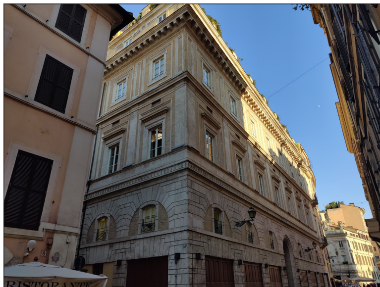
Figure 12: Raphael, Palazzo Alberini, showing an ordine contratto on the first floor of the facade, ca. 1517–1519, Vicolo del Curato, Rome. Photo by Max Wiringa, 2022.
