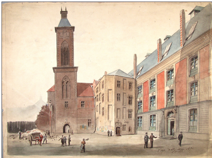
Figure 18: Edouard Boldoduc, view of Rihour during its demolition in 1857. From left to right are the 19th-century belfry, the 15th-century stair tower, and the 18th-century reconstructed wing, 1857. ML 1462, Musée de l’Hospice Comtesse, Lille. Photo by Frédéric Legoy – Musée de l’Hospice Comtesse/Ville de Lille.
