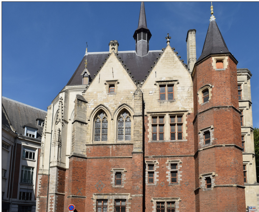
Figure 1: Palais Rihour, Lille, view of the lesser chapel and ducal oratory with the chapel behind, 1462–1465. On the right, behind the smaller octagonal staircase turret, is the ceremonial stair tower, which was relocated and attached to the chapel in 1857. Photo by Merlijn Hurx, 2019.
