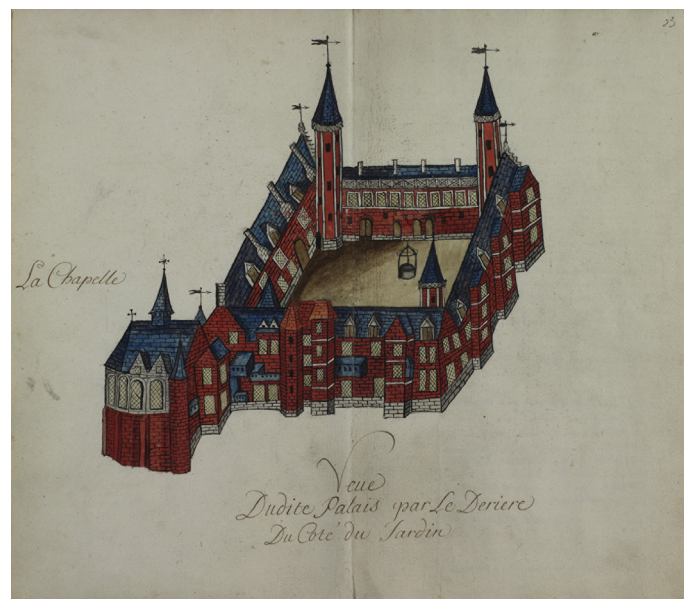
Figure 7: View of Palais Rihour from the south-west, with chapel and ducal wing in front. Immediately to the right of the chapel is the gable of the sallette , which is depicted here as being made of brick with a limestone chimney, while in reality it was dressed with stone. 17th-century copy of a 16th-century manuscript, draughtsman unknown. Ms Leber, 5903, fol. 20v-21r, Bibliothèque Municipale, Rouen. Photo by Charlotte Bosmans.
