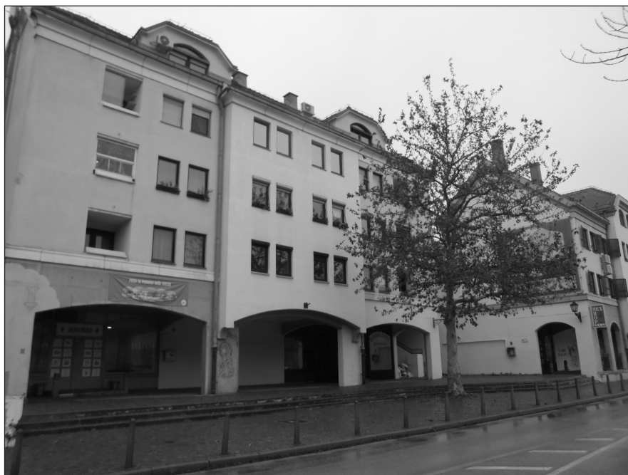
Figure 12: Jovan Milošević, building B, on Vojašniška street. Photo by Raimondo Mercadante, February 2020.
