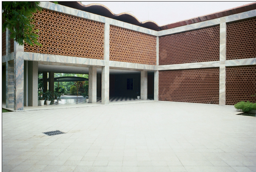
Figure 4: Satterlee and Smith, US embassy residence, Asuncion, Paraguay, 1960 (photographs related to embassies, consulates, and other overseas buildings, record group 59, National Archives, https://catalog.archives.gov/id/24260566 ).
