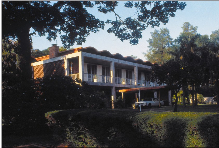
Figure 5: Satterlee and Smith, US embassy residence, Asuncion, Paraguay, 1960. (photographs related to embassies, consulates, and other overseas buildings, record group 59, National Archives https://catalog.archives.gov/id/24260580 ).
